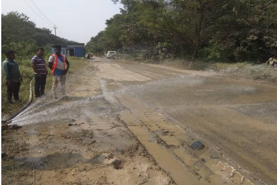
Photograph showing water sprinkling in haul road
